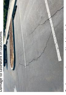
Cracks appearing on parking lot asphalt
