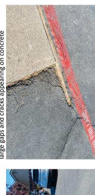
large gaps and cracks appearing on concrete
