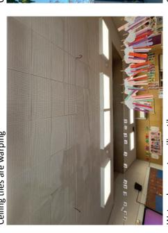
Water damage to ceiling tiles
