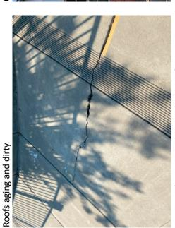
Large cracks appearing on concrete paths
