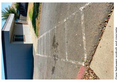
Gaps between asphalt and concrete
