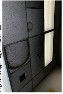
Water damage on ceiling tiles
