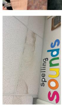
Water damage to ceiling tiles
