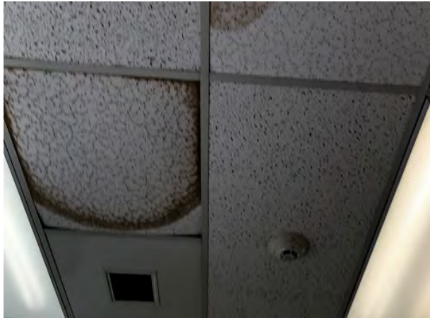
Major water damage to ceiling tiles
