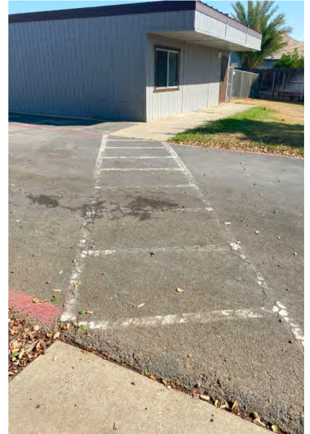
Gaps between asphalt and concrete
