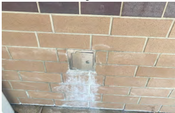
Water dripping on exterior wall leaving deposits
