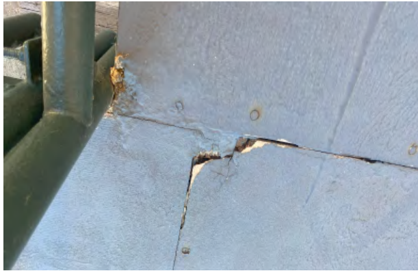
Cracks/damage to wheelchair ramps
