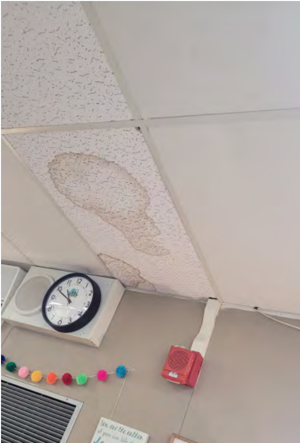
water damage on ceiling tiles
