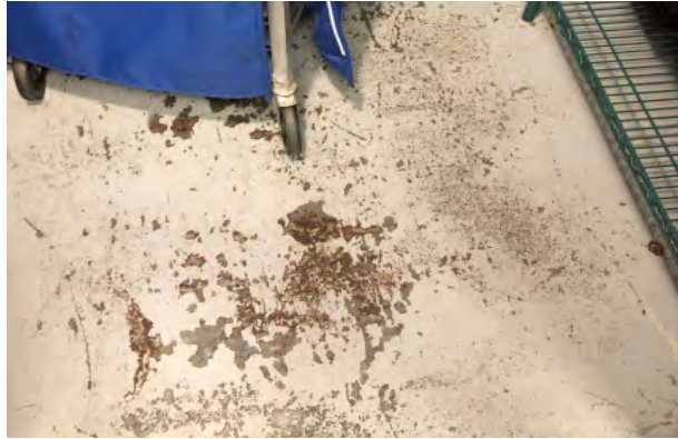
Floor damage due to kitchen equipment
