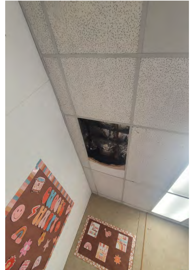
Missing or damaged ceiling tile
