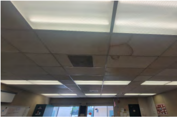
Water damage has affected the ceiling tiles
