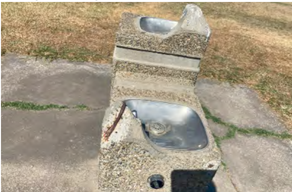
Drinking fountains are broken/damaged
