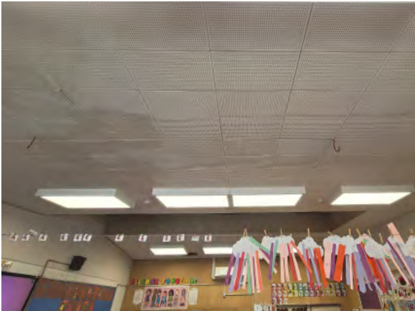
Water damage to ceiling tiles
