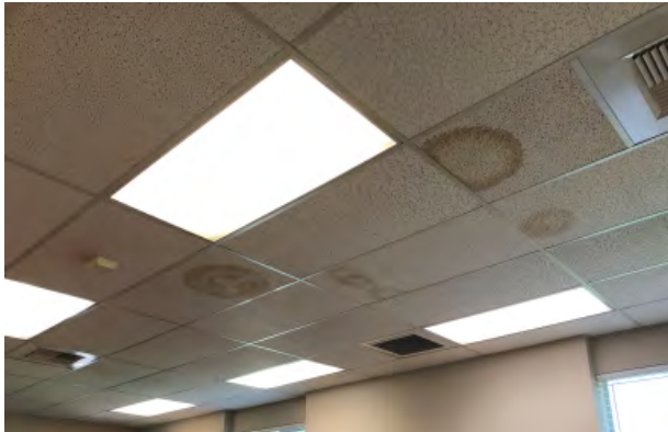
Water damage to ceiling tiles
