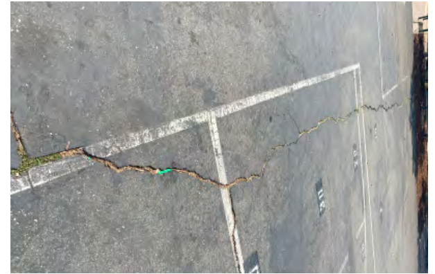
Cracks appearing on asphalt
