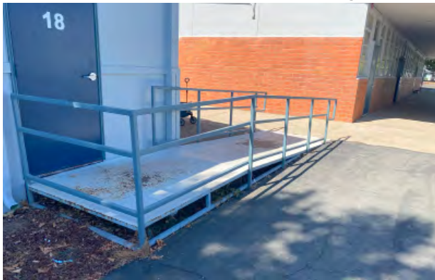
Ramps have sign of wear and tear
