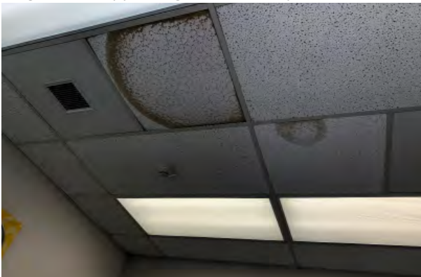
Water damage on ceiling tiles
