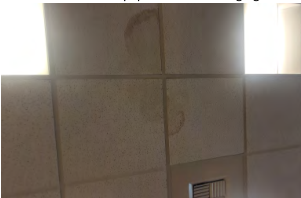
Water damage to ceiling tiles
