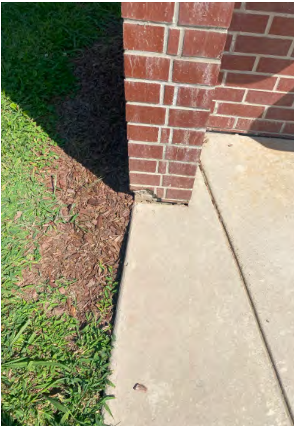
Damage to exterior brick
