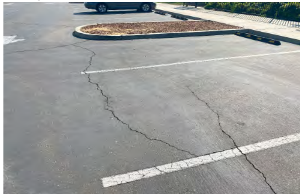
Cracks appearing on parking lot asphalt
