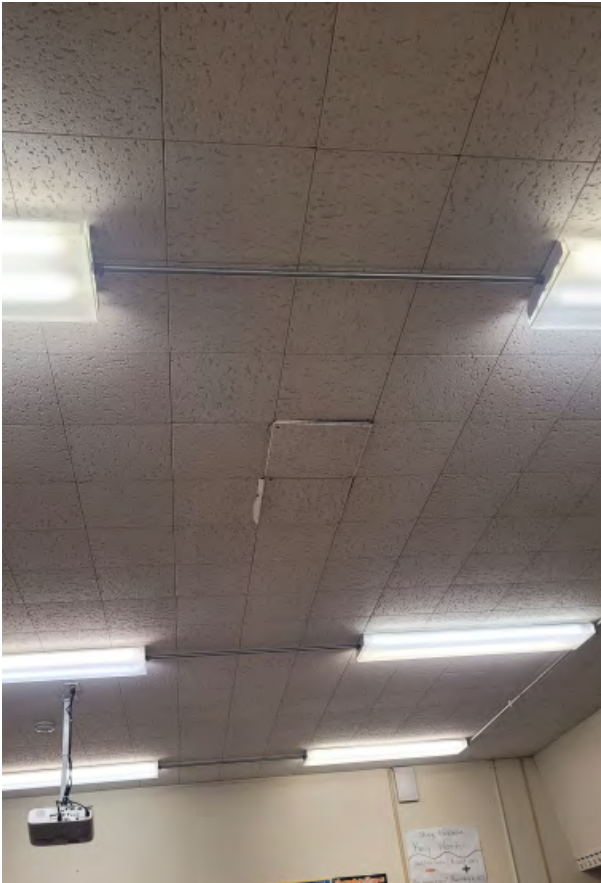
Damage to ceiling tiles
