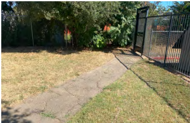
Old walkways are cracked and unlevelled
