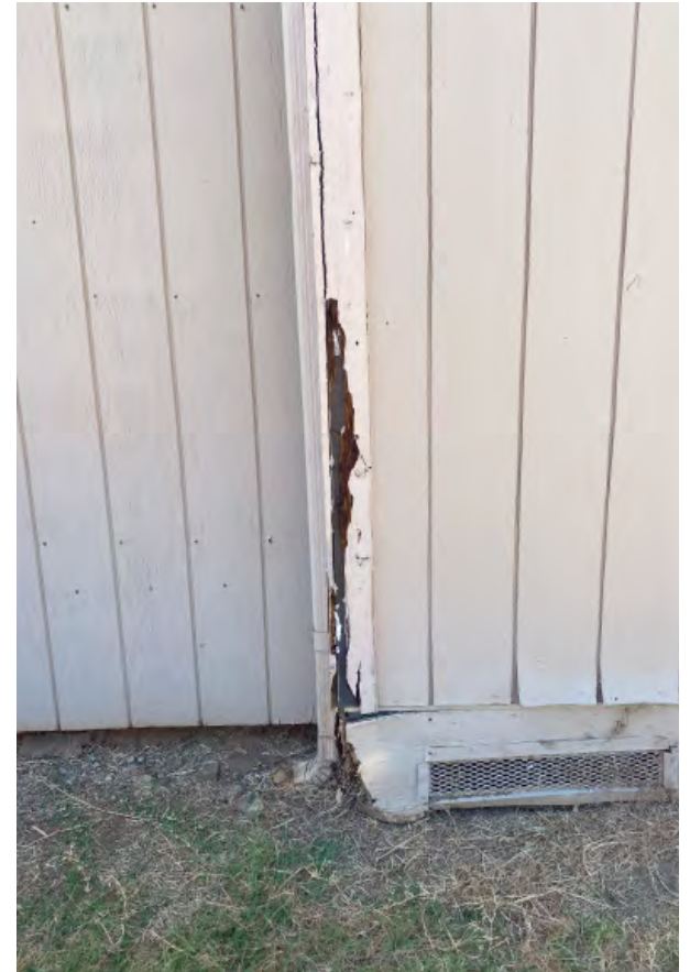
Exterior wall breaking away
