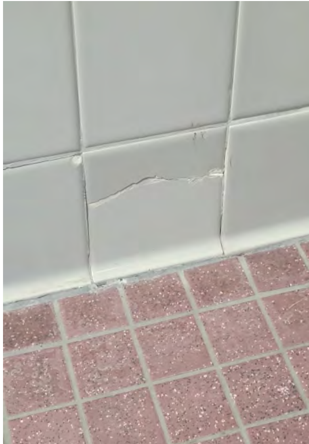
Restroom tiles are cracking
