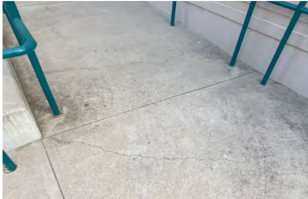
Cracks appearing on ramp walkways
