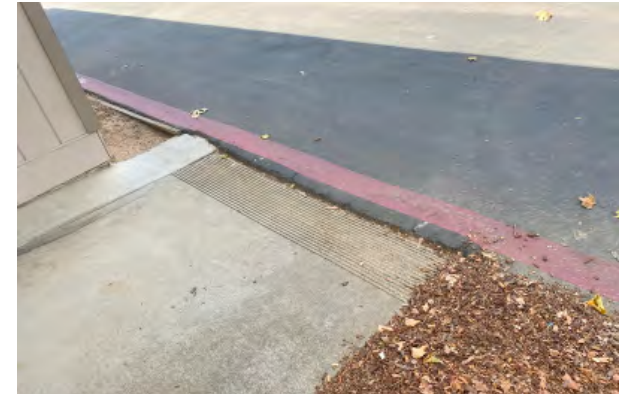
Large gaps/cracks appearing on asphalt
