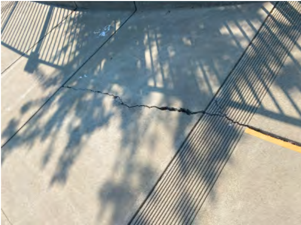
Large cracks appearing on concrete paths
